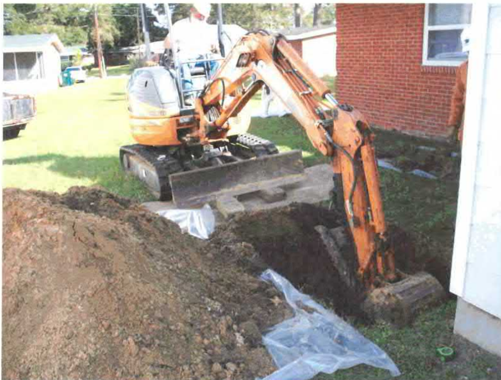
Picture 2: UST 519LaurelBB excavation in progress.
